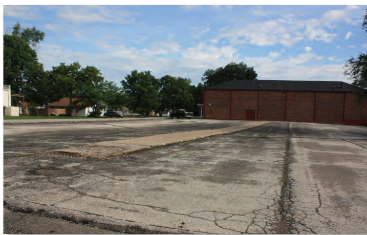
Upgrade the existing underutilized parking lot into a multi-use farmers market and commuter / downtown district / special event parking area.
