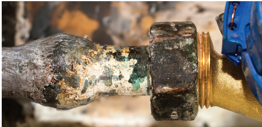
Lead pipes can usually be found in older homes, those built before 1986, according to the Environmental Protection Agency.
