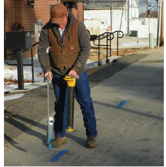
City public works crew mark water lines as part of a Kansas One-Call request.
