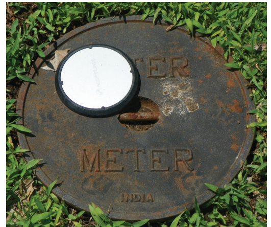
Water meter lids that are being prepped for automatic meter reader equipment.
