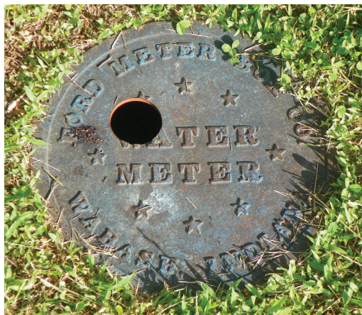
Water meter lids that are being prepped for automatic meter reader equipment.
