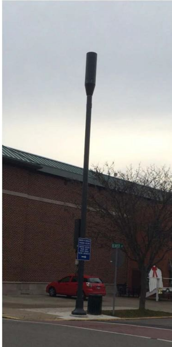
Figure 3: Replacement Pole with Attached Equipment Shrouded
